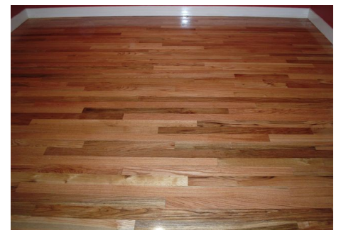
Flooring Installed in Central LA
